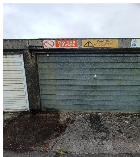
Typical door and frame showing spalling to concrete
