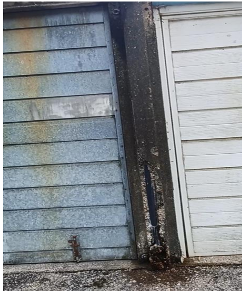
Frame detail with spalled concrete
